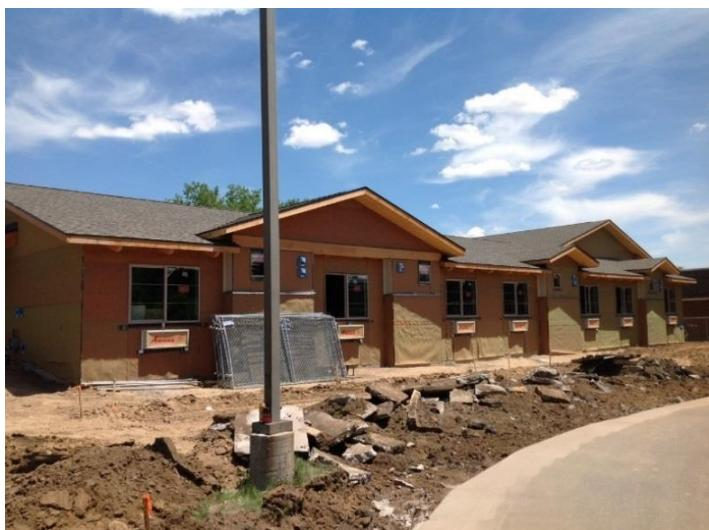
Over 10,000 sq. ft. of WrapShield RS Rain Screen with 3mm built-in drainage matrix was installed on Harvard Square Assisted Living.
