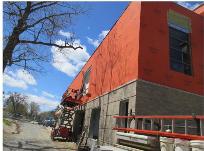
*WrapShield SA Self-Adhered was chosen because its free of harmful VOCs and no primer is required, making it safe to install on campus.*
