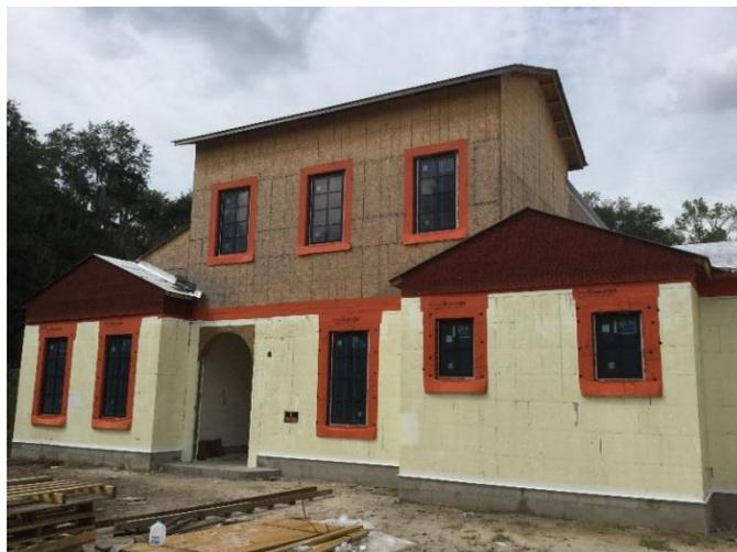
WrapShield RS Rain Screen offers an all-in-one weather resistive barrier, air barrier and 7mm rain screen drainage matrix, helping to dry out cementitious stucco and stone veneers.
