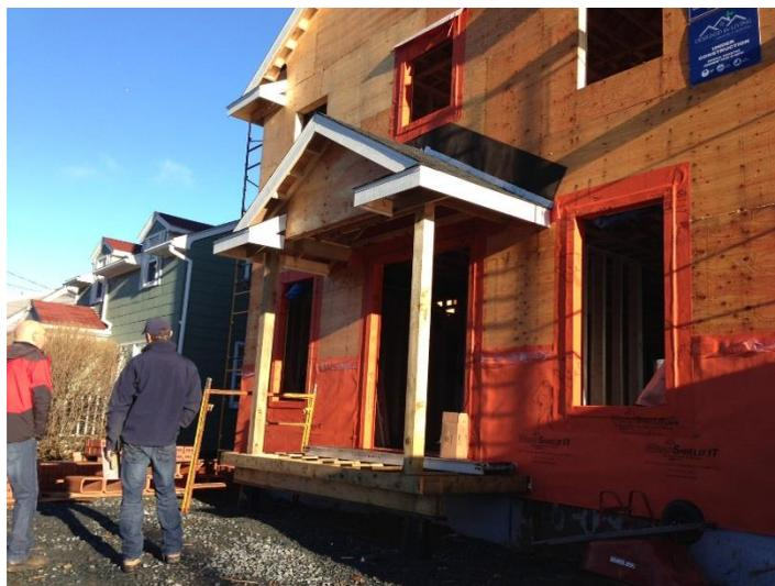
Over 3,000 sq.ft. of WrapShield Water Resistive Vapor Permeable Air Barrier Membrane was installed over plywood.
