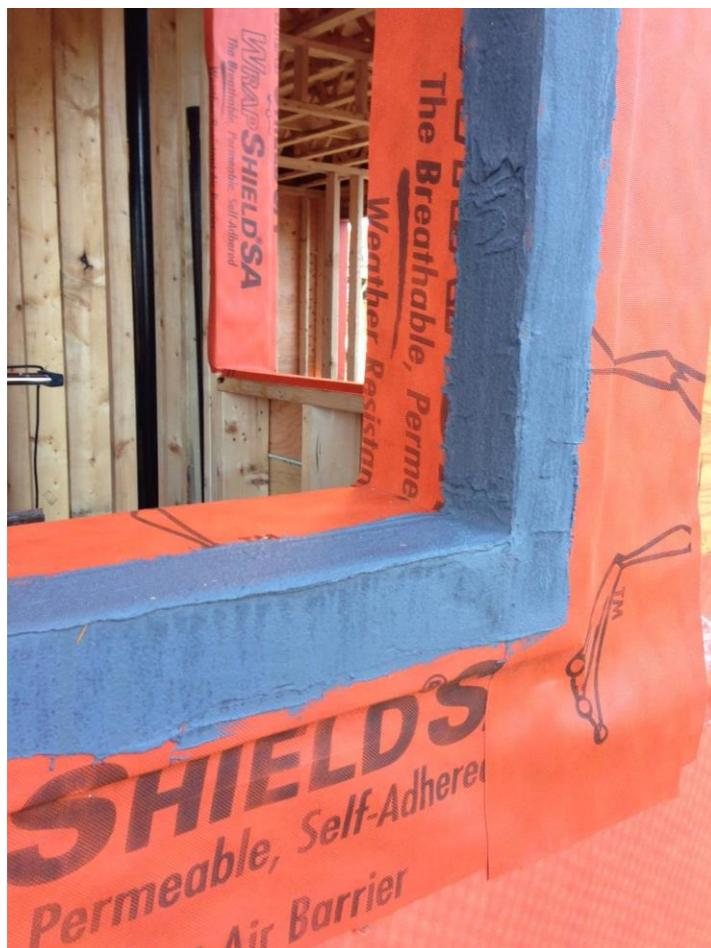
VaproFlashing and VaproLiqui-Flash were used on all window and door openings reducing installation time and ensuring breathable but air-tight seals.
