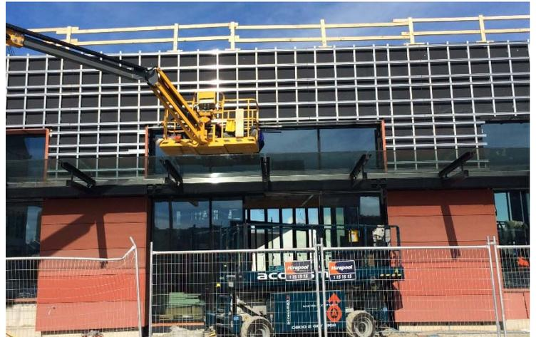
24,800 sq. ft. (2,300 m<sup>2</sup>) of RevealShield SA Self-Adhered (black) was applied in a rain screen application behind an open joint Fiber-C panel cladding attachment system (orange).
