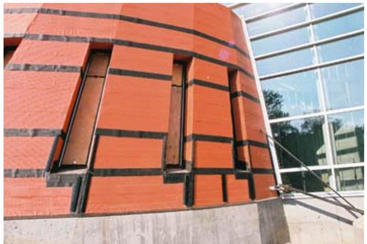
*VaproFlashing Black was used for the open joint cladding.*
