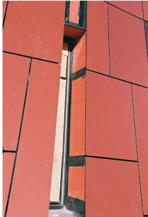
Above: Window waiting for fixtures and glass, remaining cladding will be installed after window is completed..
