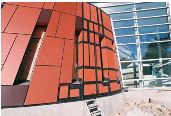
*Left side of image shows cladding installed, right side WrapShield SA with VaproFlashing Black for the 1" open joints.*
