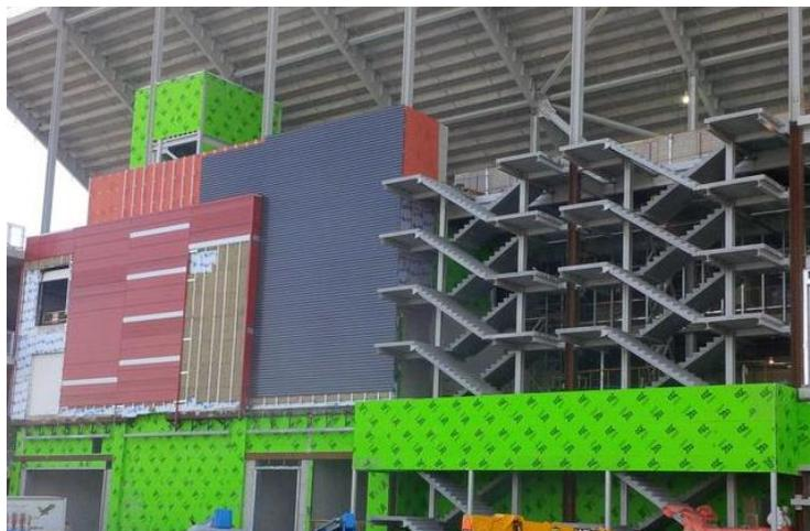
No primer is required with WrapShield SA Self-Adhered, which avoids costly delays due to primer application restrictions.
