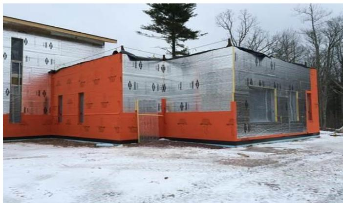
The Bear Creek Community Charter School in Pennsylvania was installed with roughly over 30,000 sq. ft. of WrapShield SA Self-Adhered Water Resistive Vapor Permeable Air Barrier Membrane, which was adhered to Dow Thermax™ Foil Faced Polyiso Sheathing.
