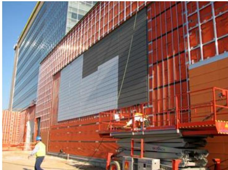
Over 40,000 sq.ft. of WrapShield Water Resistive Vapor Permeable Air Barrier Sheet was installed on the new Edward Jones building as part of their headquarters in St.Louis.
