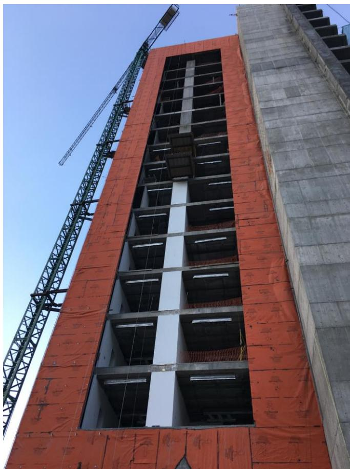
*Approximately 30,000 sq. ft. of WrapShield SA Self-Adhered Water Resistive Vapor Permeable Air Barrier Sheet Membrane was installed in the construction of Alpino Condo Tower.*
