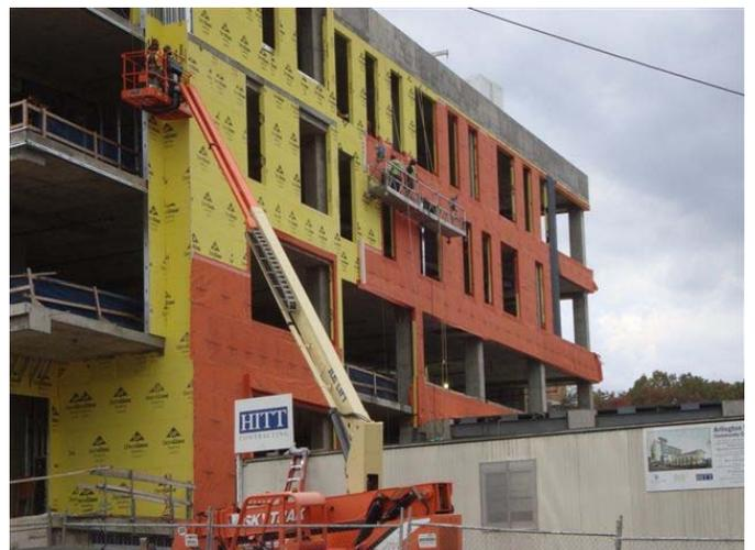
Over 56,000 sq. ft. of WrapShield Water Resistive Vapor Permeable Air Barrier Membrane Orange was installed.
