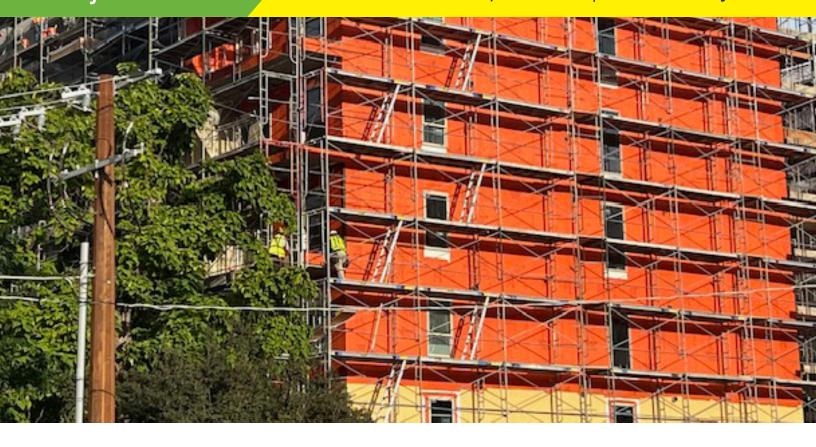
DeWitt Apartments, nestled in the heart of Salt Lake City, installed over 80,000 sq. ft. of WrapShield SA Self-Adhered on a plywood substrate.
