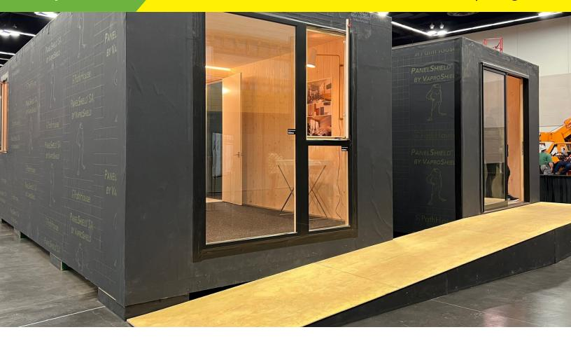
VaproShield is pleased to partner with PathHouse, whose objective is to provide the nation, starting with the Oregon region, with affordable housing. PathHouse is a modular mass timber housing system. These unique homes use both PanelShield SA weather resistive air barrier on the walls and SlopeShield Plus Self-Adhered roofing underlayment.
