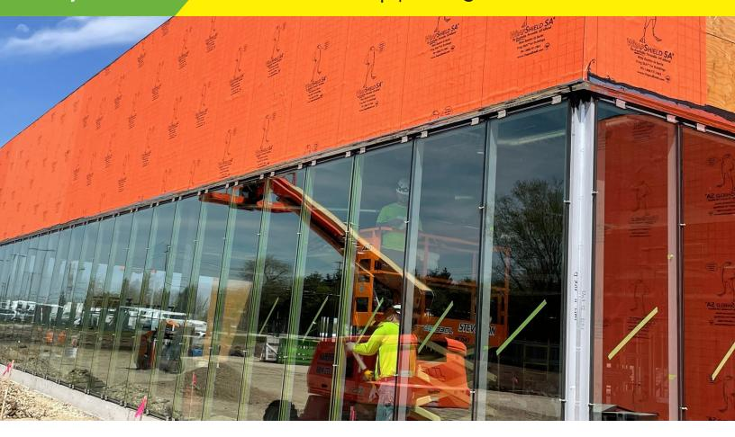
Over 10,000 sq. ft. of WrapShield SA Self-Adhered Water Resistive Vapor Permeable Air Barrier Sheet Membrane was installed in the construction of a state-of-the-art Cadillac Dealer in Barrington, IL.
