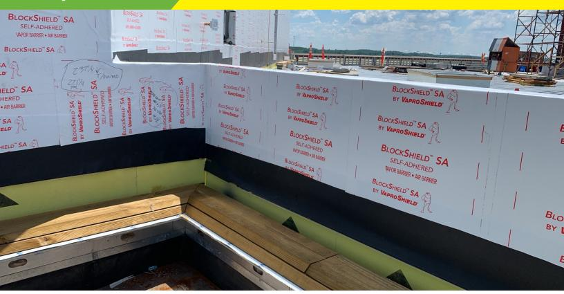
The new Gerald R. Ford International Airport expansion project used over 40,000 sq.ft. of BlockShield SA over gypsum sheathing plus VaproShield flashing accessories: BlockFlashing and VaproBond. BlockShield SA is a non-asphaltic air water and vapor barrier that offers an aggressive pressure-sensitive adhesive and 12 month UV and climate exposure, the perfect choice for Michigan's ever-changing weather.
