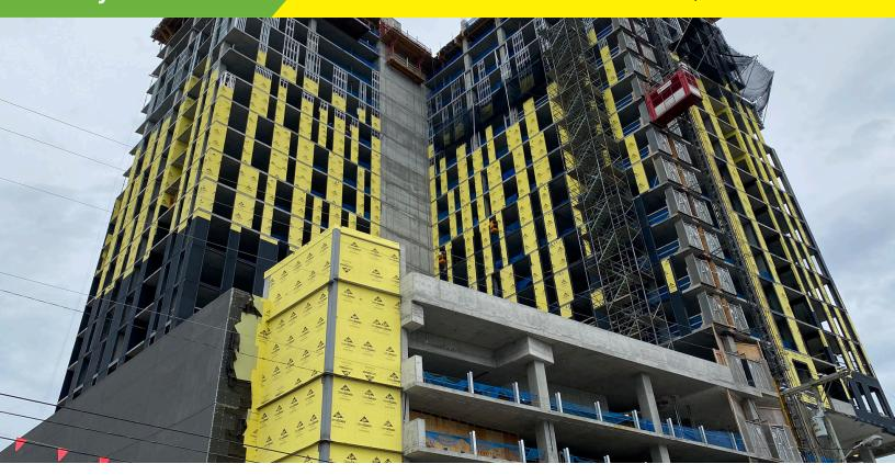
The 29-story urban apartment building was erected in Nashville's "SoBro" neighborhood used 200,000 sq. ft. of RevealShield SA, WrapShield SA, and accessories to provide a protective WRB and air barrier under the ACM (open joint) cladding. For this premier mixed-use project, the architect selected a combination of WrapShield SA, RevealShield SA, and the VaproLiqui-Flash system for its easy installation, superior UV-stability, and water holdout.
