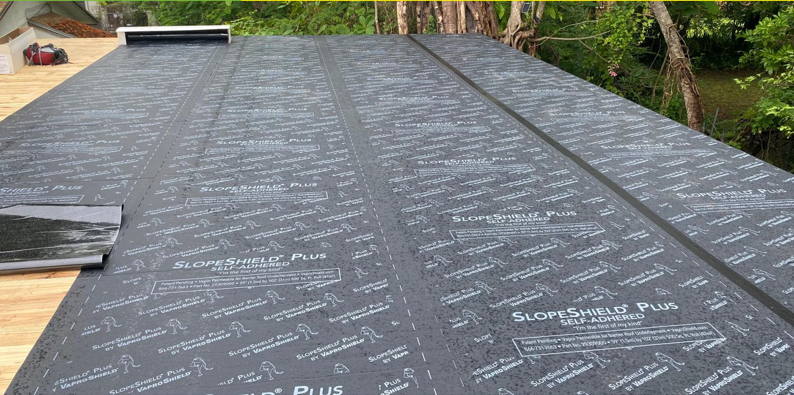
Over 3,500 sq.ft. of SlopeShield Plus Self-Adhered (SA) vapor permeable roofing underlayment was used in the first cross-laminated timber (CLT) project, Grovehaus, in Miami, Florida. In addition, 3,300 sq.ft. of PanelShield SA, a permeable polyester air barrier WRB membrane, was used on the exterior walls in this mass timber build.
