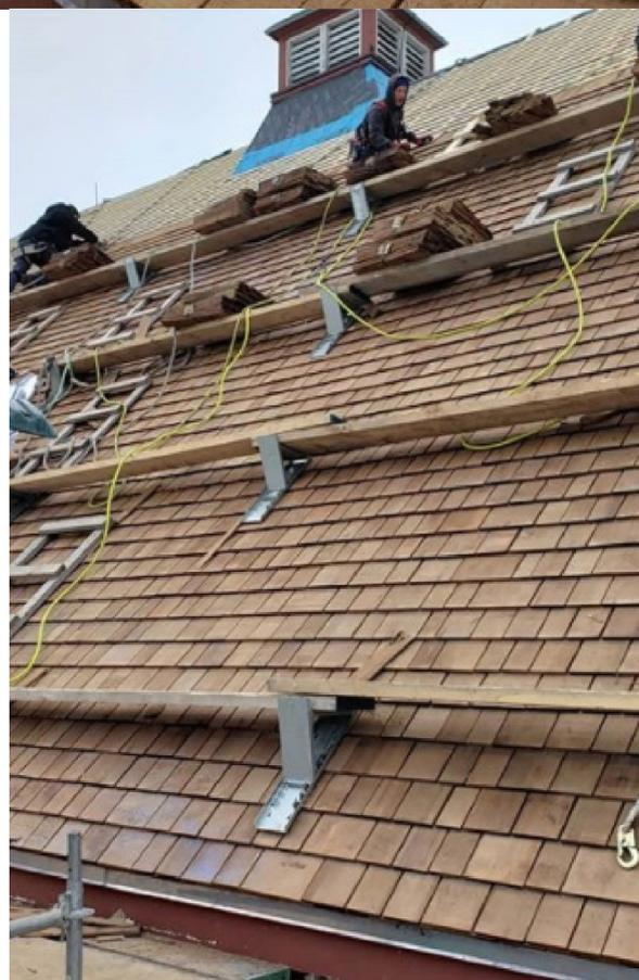
SlopeShield Plus roofing underlayment installed under cedar shakes.
