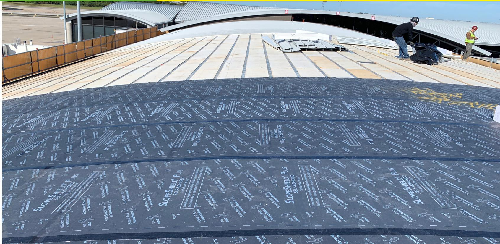
Over 120,000 sq. ft. of SlopeShield Plus Self Adhered was installed over existing roofing materials at the Tampa Airport, HCAA Project No. 6545 19 TPA Airside F Re-Roof. One of the key reasons the Architect chose SlopeShield Plus SA was its **ability to breathe** (due to its permeability), drying any moisture that would occur between the existing roofing material layers.
