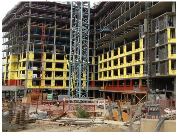
WrapShield SA Self-Adhered was installed on the new Washington Gateway mixed-use building.
