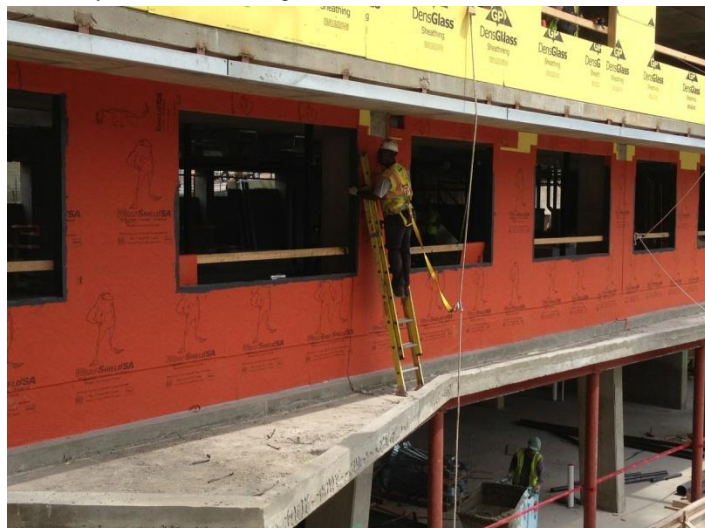
WrapShield SA Self-Adhered is phase construction friendly and does not require any special installation equipment.
