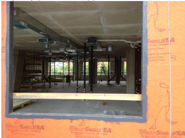
VaproLiquiFlash was used around the window openings.
