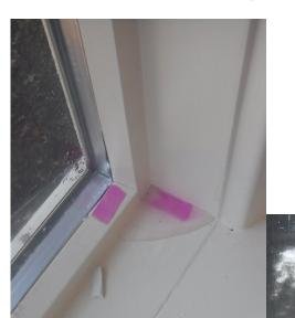
The home's windows were suspected to be a contributing factor for additional moisture damage, so the consultant performed window spray tests to confirm the leak sources. Three window units were identified as leaking and were removed and replaced.
