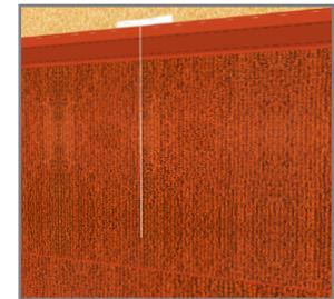
7. Lay original flap of WrapShield RS onto adhesive area of WrapFlashing SA to complete the joint. Place min. 2 staples in top 2" of each flap above tape line.
