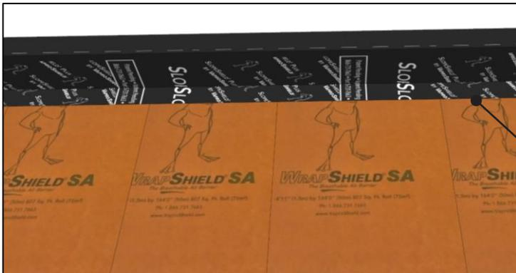
**Step 2: Install SlopeFlashing around eaves, shingling over wall membrane**
